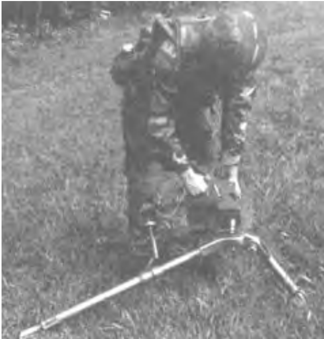
Figure 5-51. Mounting the Cradle on Tripod.
